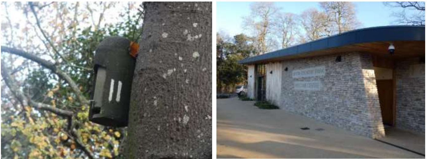
Fig 10 Artificial bat roosts: Left: bat box in the Grove; Right: Upton Country Park’s new Welcome Centre has gaps in the soffit to allow bats to enter and the gaps in the stone walls could also provide roosting spaces.
