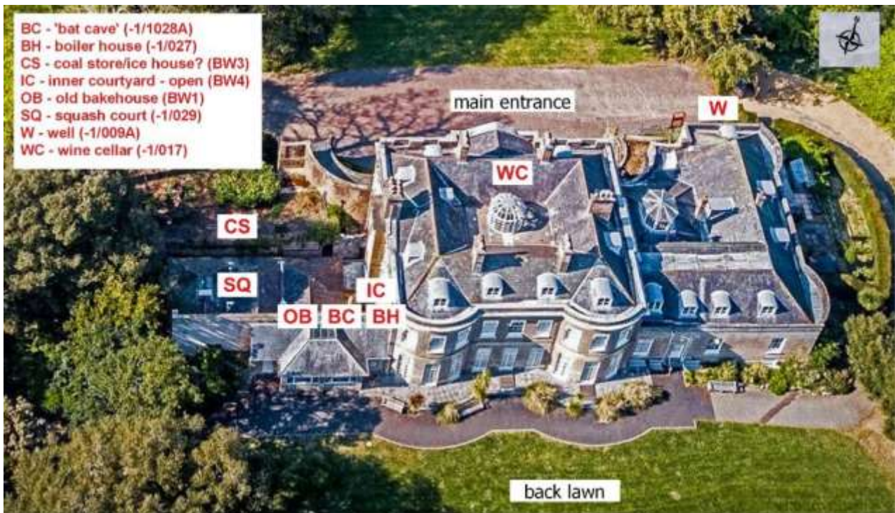
Fig. 6 – Aerial photo of Upton House indicating approximate location of rooms in the basement. Room names and numbers are as used by the Council’s Property Services Department and/or in the 2010 Conservation Management Plan 5 , except for the ‘bat cave’ which is usually un-named on plans.
